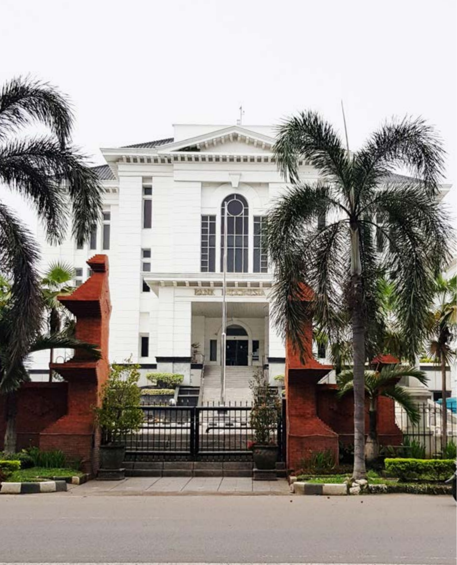
The Bank Indonesia building in Kelurahan Lemahwungkuk. Asian Development Bank.
